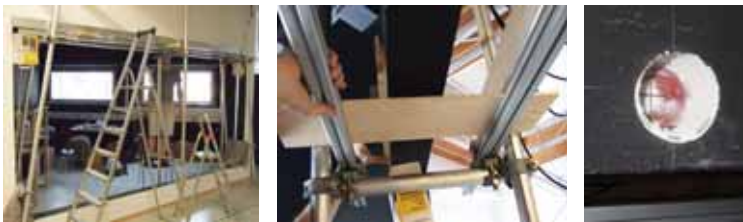
Figure 2.35: To attach the screen to the frame, we drilled holes in the screen and the frame. Here, preparations are shown for drilling the holes. It was a challenge to be accurate enough.
